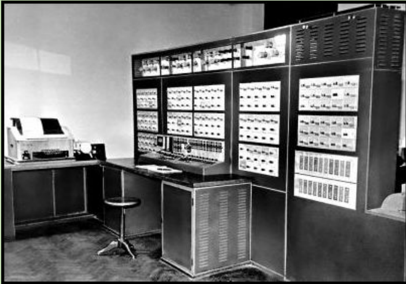
Setun Balanced Ternary Computer (Mosow State University 1958)
